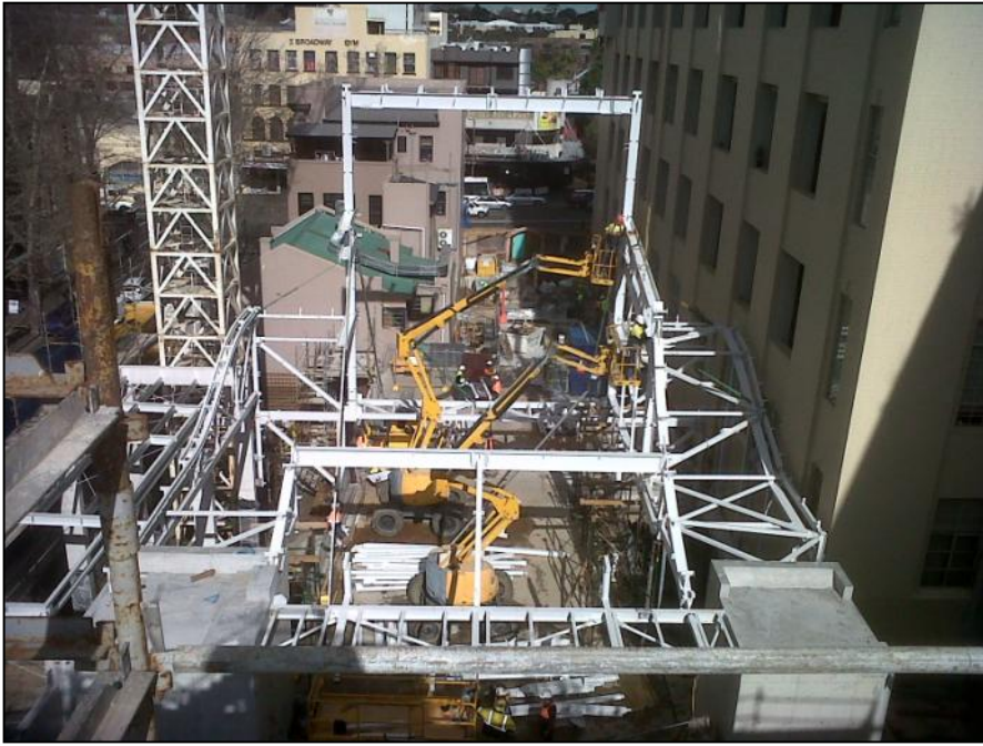
The construction of the framework for the building.
