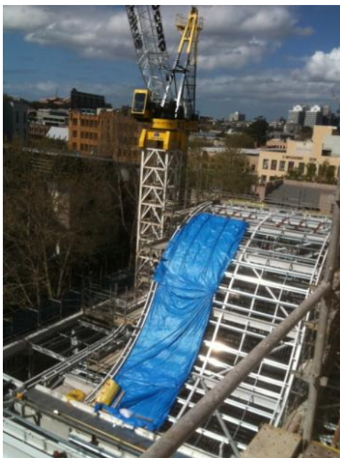
Raising the Roof—the New Barneys begins to take shape.
