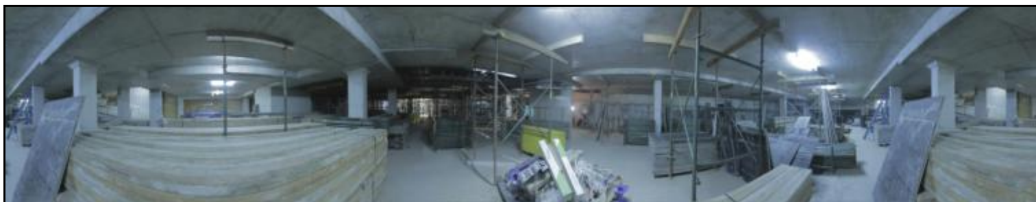
Panorama of the basement level of the new building at Broadway
